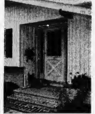
INTERESTING architectural effects may be achieved with solid vinyl-V-grooved vertical siding accenting highlight areas, such as doorways, porches, porch ceilings or gable ends of homes. It is often specified for the lower sections of garrison colonials. From Bird & Son, Inc., East Walpole.
